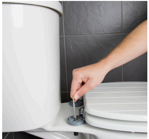
FIX - Position the seat, press the hinges in place and tighten the fixing bolts for a sturdy no slip installation.
