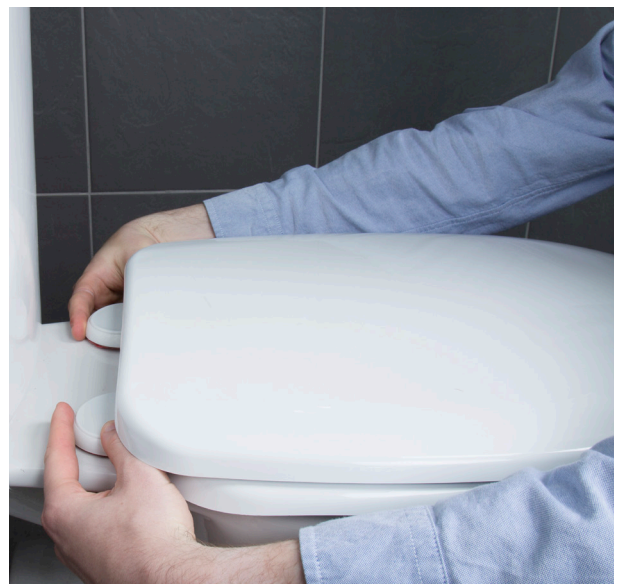
FIX - Align the hinges to the toilet pan and push hinges in place.
